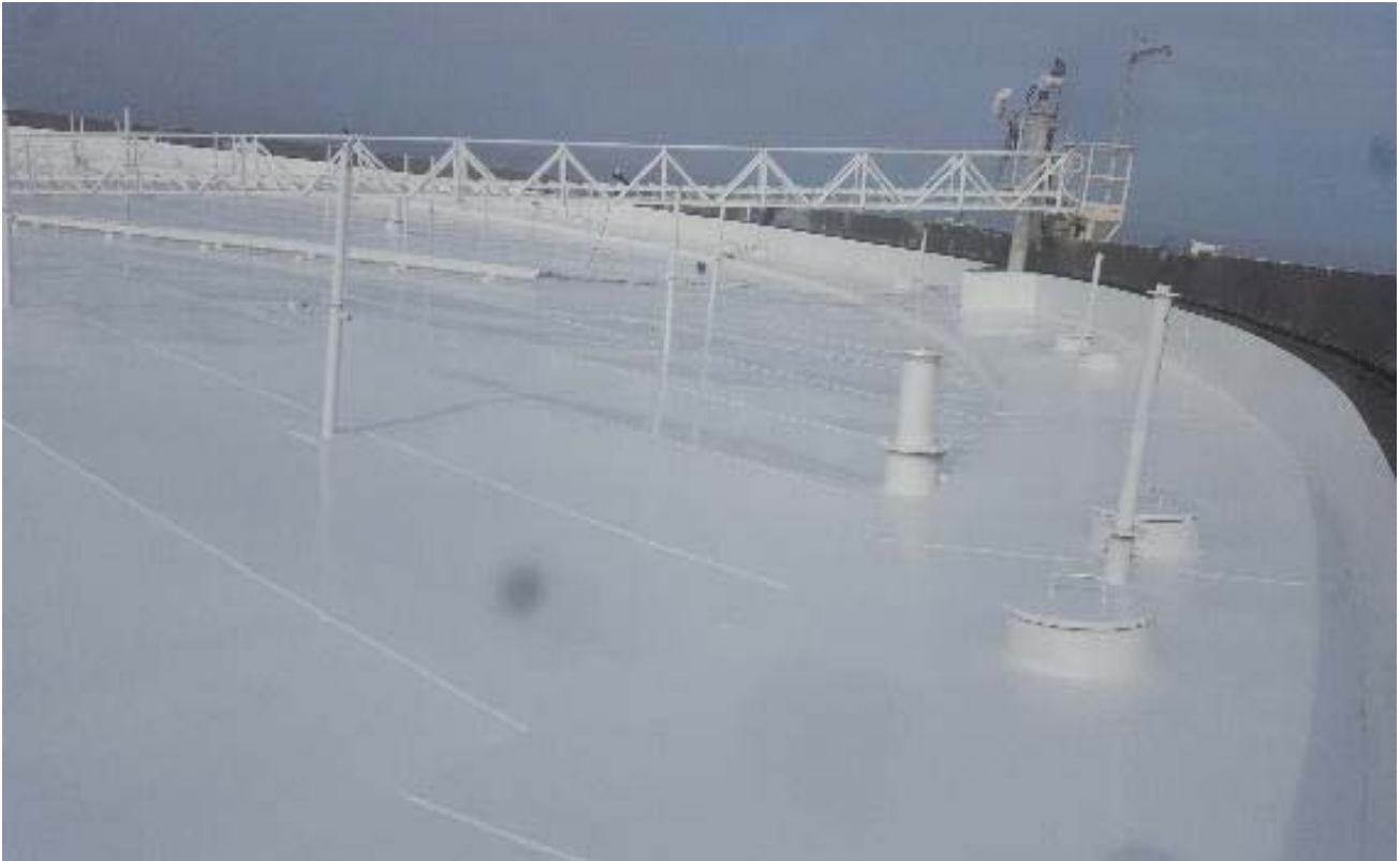
Floated roof appearance after polyurethane top paint
