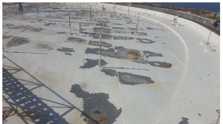
Floated roof initial condition
