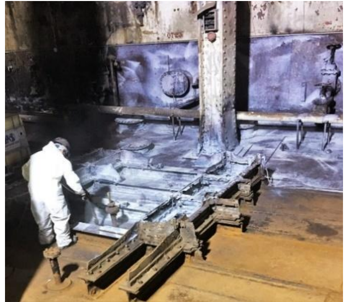
Corrizon Base application inside the boiler room
